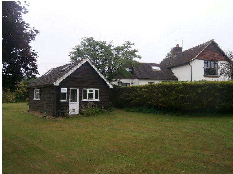
Photo 2. Existing building viewed from the southwest.
