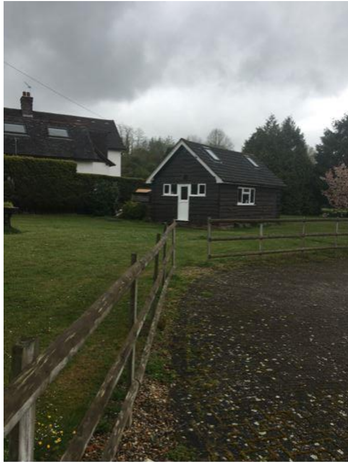
Photo 1. Existing building viewed from Walnut Tree Cottage the northwest.
